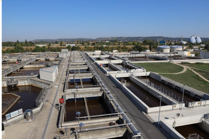
Expansion Aeration Plant, 2. Lot
